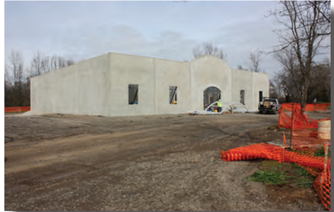
Walls are up
