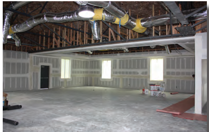
Board room and offices are coming along
