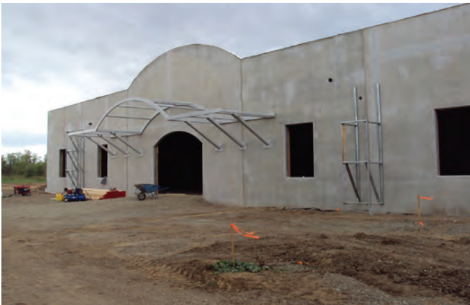
Awnings installed and the roof is on
