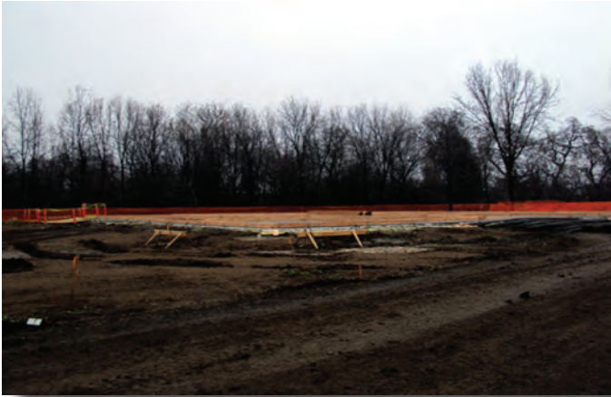
Foundation is ready
