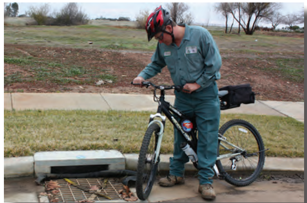
Checking Storm Drain for standing water
