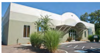
New Chico Substation
